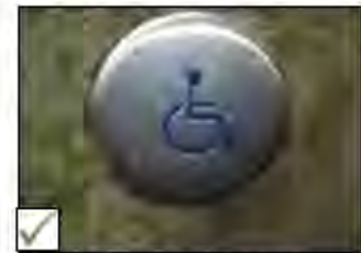
Example of circular power door operator control.
