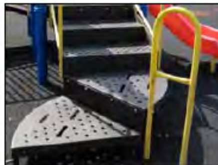
Transfer system to connect elevated play components.
