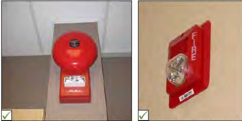
Example of combined visual and audible alarm signals. Public facilities should have both visual and audible fire alarm systems strategically located.
