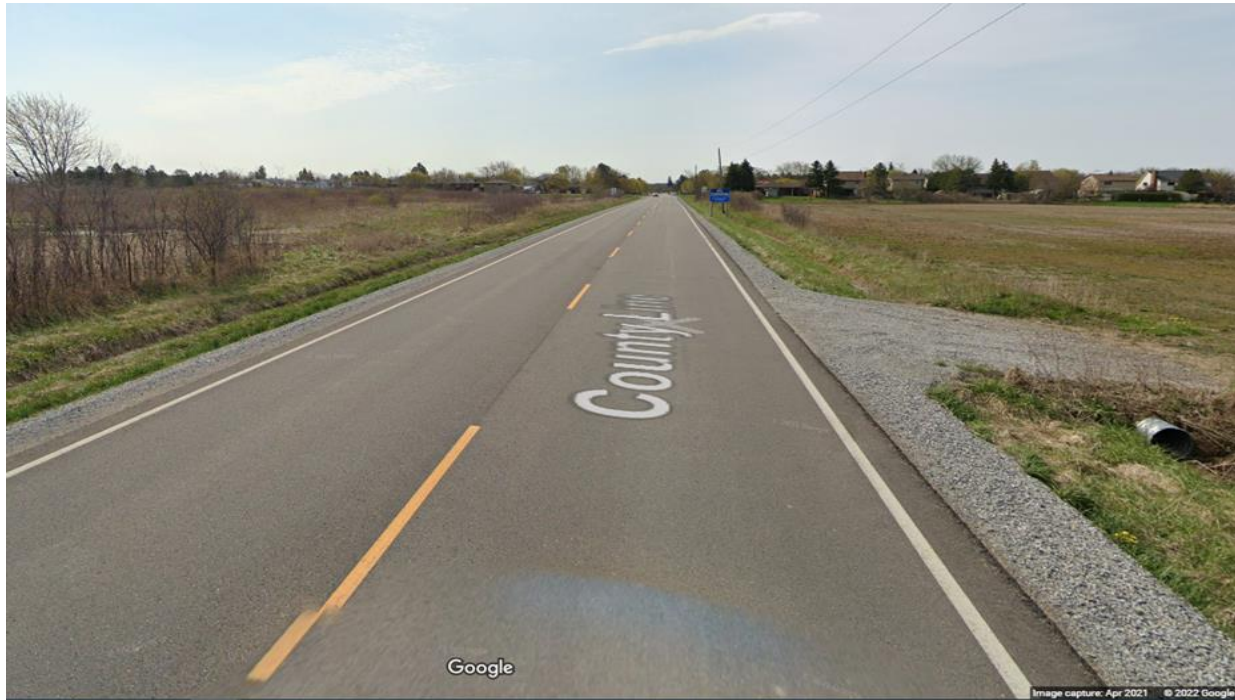
Figure 16: Marshall Road – LCB Rural (Fair PCI=41)
