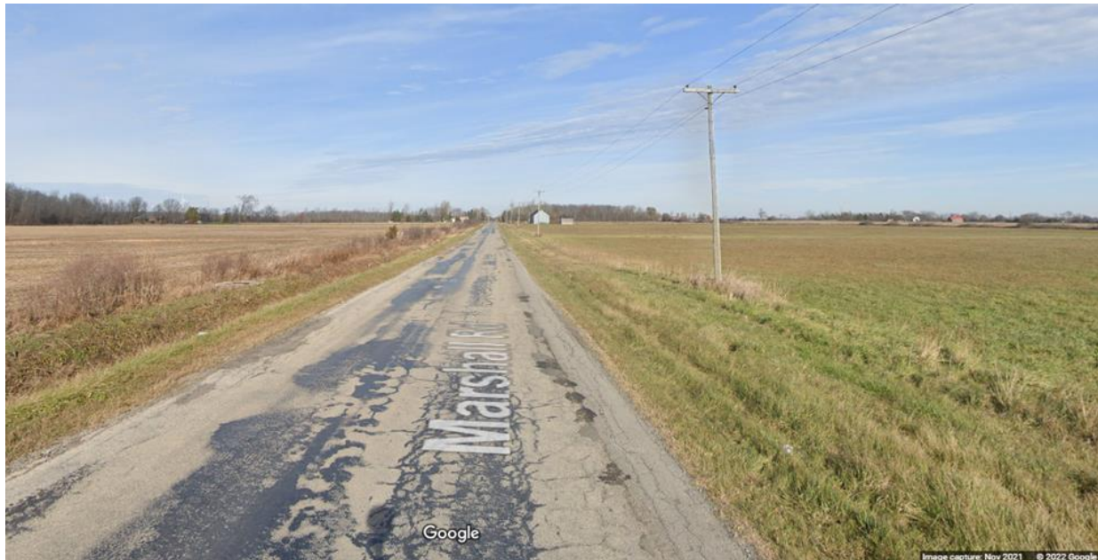
Figure 16: Marshall Road – LCB Rural (Fair PCI=41)
