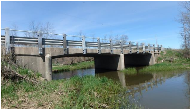
Figure 26: Lakeshore Road Culvert (BCI=87 Very Good)
