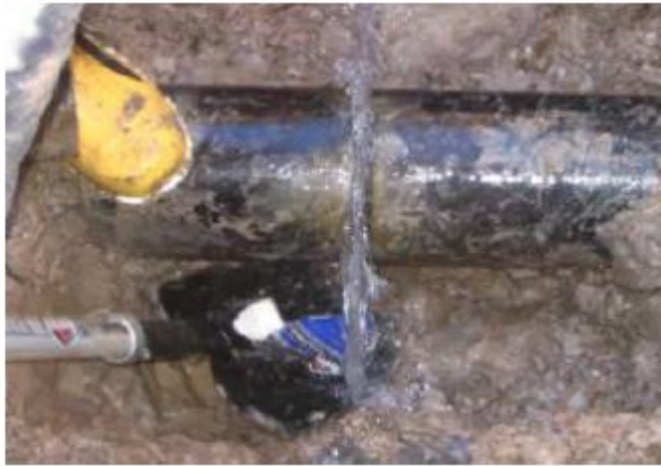
Figure 1: Circumferential watermain break with flow maintained until after an Air gap was created.
