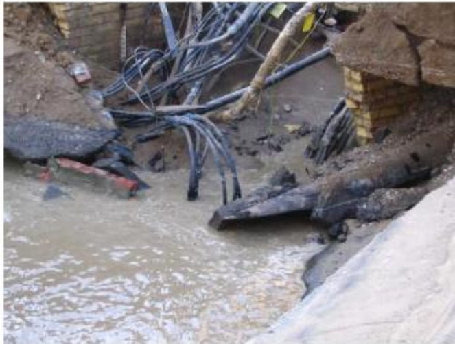
Figure 4: Spiral watermain break with evident Contamination.
