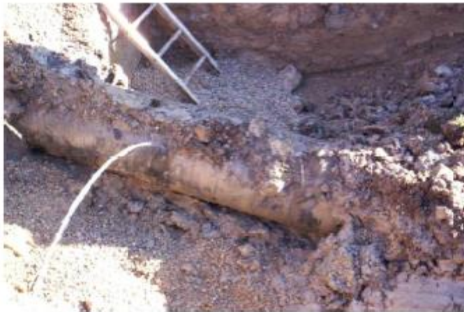
Figure 2: Corrosion hole leak in a watermain with flow maintained until after an Air gap was created.
